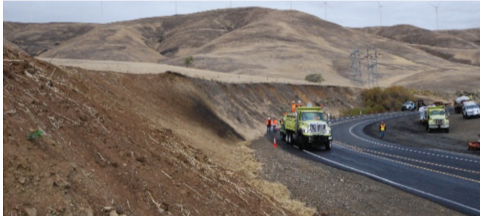
Initial installation - notice the severely arid conditions.
